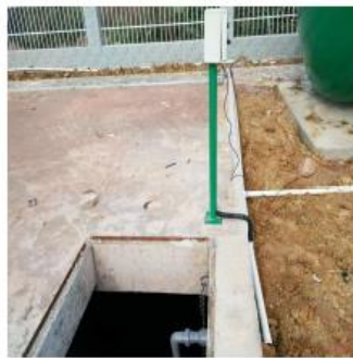
Figure 7: Installation Standards Diagram for Lift Pump Control
