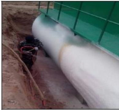
spray insulation coating
