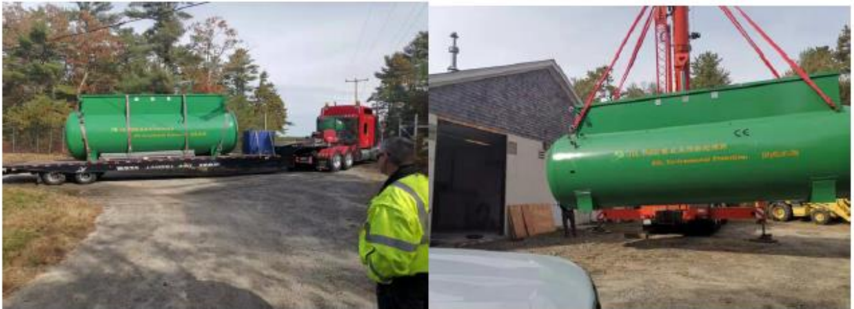
The site installation of FMBR equipment
