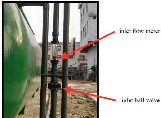
Figure 2: Installation Position Diagram for Flow Meter and Inlet Valve
